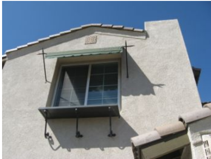
Exterior Areas Eaves & Facia
