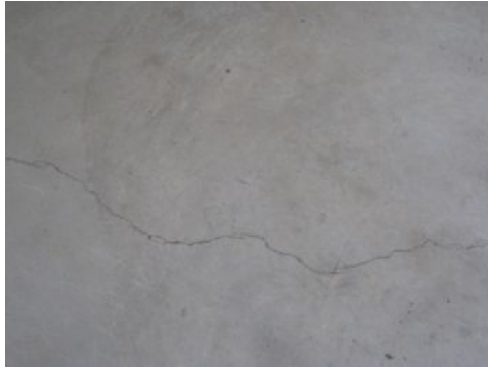
Grounds Driveway and Walkway Condition
