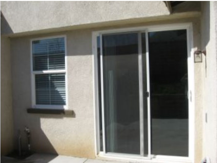
Exterior Areas Stucco
