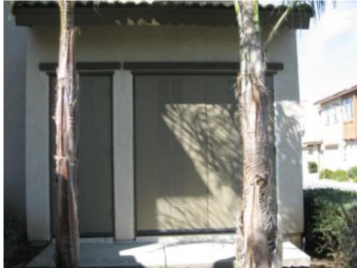
Exterior Areas Doors
