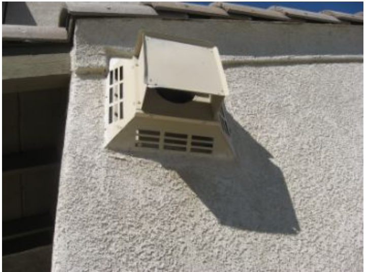
Exterior Areas Stucco
